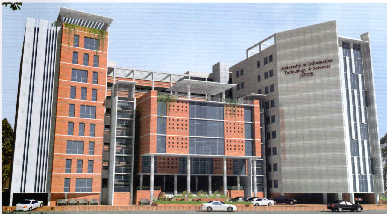
The Under construction Proposed permanent campus of UITS
